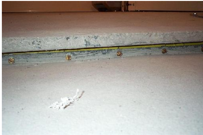
Figure 1. Water nozzles used to wash the manure from the gutter portion of the pen.
